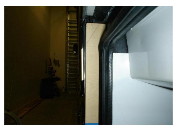
This is what the left end of the door looks like after my three wooden block modification. You can see the 3/16 inch gap which TMH built into the wall. There is no way to correct this in my opinion without major work by TMH.
