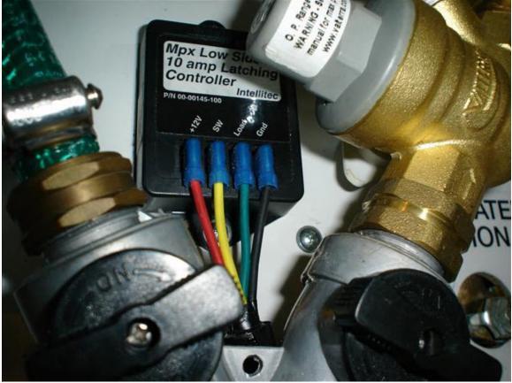
These four connections are the four wires we are most concerned with. The Red is +12VDC, the Yellow is the Switch (SW), the Green is the Load and the Black is the ground. If you are having problems with your water pump, I suggest you move this Low Side Latching Controller to a place convenient for troubleshooting, now and for the future.
