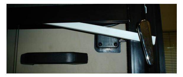
After the spacer was removed I was then able to lift the glass upward move the bottom of the glass out of the bottom track and remove the glass from the metal frame.
