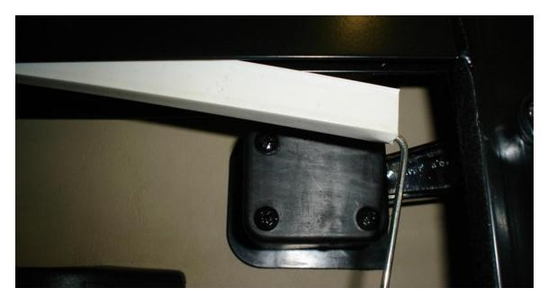
As you can see the white plastic spacer does not extend the full length of the upper or lower tracks. I hooked the spacer pulled it down and slid the spacer to the right until I could completely remove the spacer from the track. Looking at the following picture you can see how I slid the spacer between the screen door handle and the screen door metal frame to remove it. I did not want to exert too much bending pressure on the plastic to prevent damaging it.
