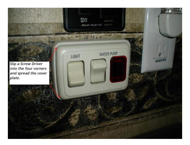
After slipping a screw driver one corner at a time into each of the four corners the cover should slip off. Make sure to be gentle or you will damage the plastic prongs which mate with the four holes on the switch plate.
