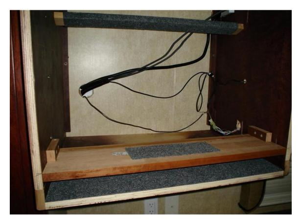
The above picture shows the installed 3/4 inch cherry stained hardwood shelf with a back attached. After assembly a small cabinet is formed which is used to store the remote controls when they are not in use. Note the installed felt pad in the center of the shelf it was placed here to prevent the plywood mount from making noise after the TV is installed and while traveling down the road.
