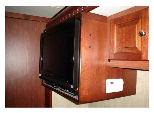
We used a cherry trim strip around the cabinet face to finish off the cabinet stained to match the Cherry Bark color. Note the hardwood plugs in side of the cabinet. Below is the finished TV cabinet with the new 26" LCD TV.
