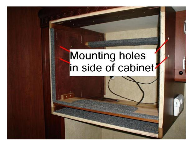
Felt was glued around the edge of the cabinet where the TV may have rubbed which would have made noise while traveling. Note the addition of the two holes on both sides of the TV cabinet. Screws will be installed in these holes from the outside to retain the TV in its cabinet. The holes were counter sunk in the cabinet to allow the installation of Cherry Bark stained hardwood plugs, the same plugs removed from the original OEM TV trim ring.
