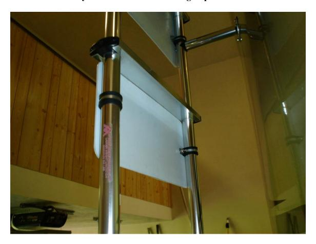
My ladder rails are 11 5/16 inches from center of rail to center of rail. I always use stainless steel hardware. When I finish a project I desire for the project to always be finished. I do not like to rework a project due to having used inferior parts.
