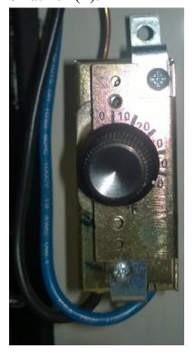
The thermostat shown to the left has been used by Tiffin for many years it's the only thermostat I've seen used on Tiffin coaches with Aqua-Hot's basement heating system.
