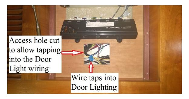
As show in the above photo, an access hole was cut in the hidden panel allowing me to tap into the door light wiring. After tapping the two new wires were routed into the next compartment where I was able to access a hole Tiffin had drilled thru the outside wall of the coach to route the power leads for the door awning. After removing the top half of the panel I was able to access the inside coach wall where Tiffin drilled thru the wall to route the awning wiring.
