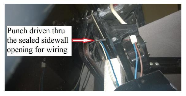
Finally able to push a twin lead 22 gauge zip wire thru the hole where the wiring was connected to a 48 inch section of high intensity LED lighting. The twin lead zip wire was carefully attached to the top of one set of awning arms with aluminum foil tape to prevent damage to the wiring when the awning was opened or closed.
