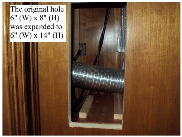
After cutting the access hole four pieces of  $\frac{3}{4}$ " x 1" wood were glued between the two panels, wood clamps were installed until the glue had dried. A piece of  $\frac{1}{4}$ " hardwood was cut 8" x 16", sanded edges beveled then stained to serve as a access cover for the dryer vent cavity.
