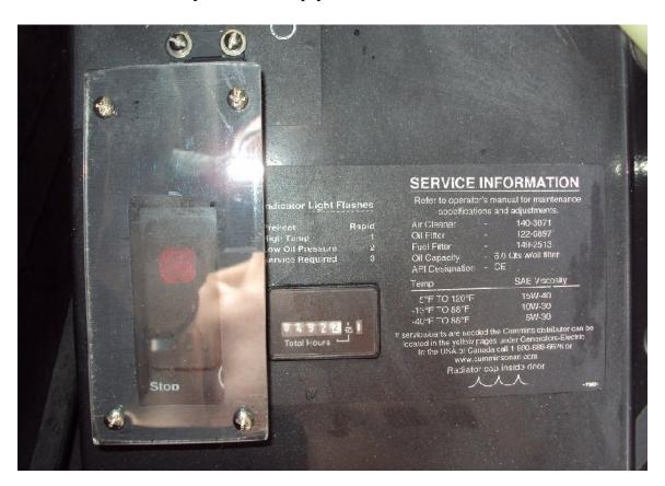
The status of the switch and its internal light can be checked by simply looking thru the cover or the generator can be started or stopped by lifting the protective cover thus allowing access to the start-stop switch.
