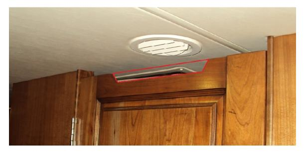
As seen in the above photo, the center portion of the door outlined in RED was removed to allow more air to flow into the bathroom from the hallway ceiling supply vent. Cutting the top of the door as shown above did not lose any strength in the door panel's construction.
