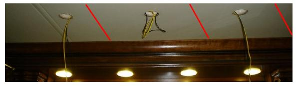
There are three structural members in this portion of the ceiling two of them are located between each of the new fixture locations the third member is located between the closet and the new fixtures. The structural members are denoted by the **RED** lines in the above photo. Those members are located on 16" centers at least in the area of this ceiling modification.
