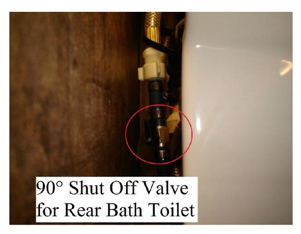
As seen in the above photo to turn OFF the water to the rear bathroom toilet requires the person to reach behind the toilet and turn the black handle 90  $^{\circ}$  to turn OFF the water to the toilet. The valve was inserted as high on the PEX supply line as possible making reaching over the back of the toilet to
