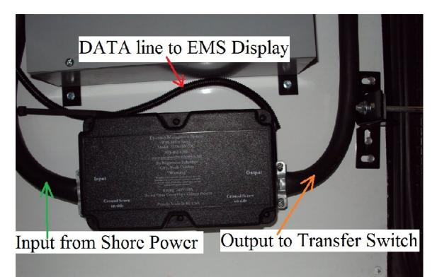
The input power cord was moved from the Tiffin transfer switch to the input side of the EMS-HW50C. A short piece of cord approximately three feet was purchased from an electrical supply house the cord has three # 6 wires and one # 8 wire. That cord was connected to the output side of the EMS and wired into the Tiffin transfer switch. The Progressive supplied **DATA** line
