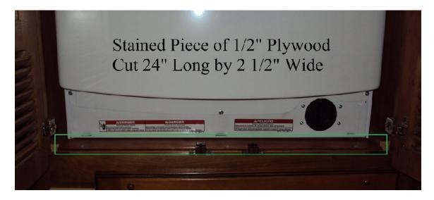
Prior to installing the plywood was stained to match the coach's interior woodwork.
