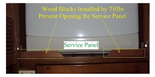
After a few measurements were taken it was decided to replace the two wood blocks with a  $\frac{1}{2}$ " thick piece of plywood cut 24" long by 2  $\frac{1}{2}$ " wide.
