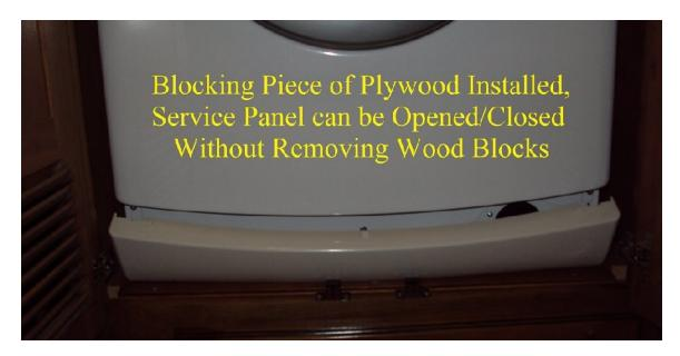
As seen above and below after the piece of blocking plywood was installed using three screws it is easy to open/close and remove/install the washer's front service panel. Time was taken to move/straighten the wood blocking at the rear of the washer thus permitting centering the washer in its closet.
