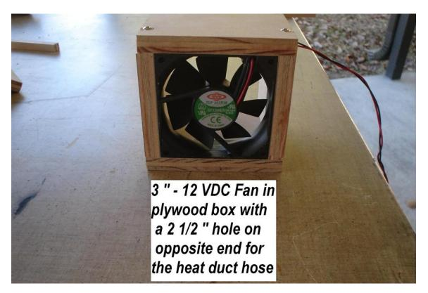
A plywood box was built to house the above fan. A cover with a 2 1/2 inch hole was attached to the back of the box this hole allows the heater hose to pass through and also to be attached to the box. 12 VDC wiring was routed from the cozy heat exchanger fans to the new half bath fan. When the Aqua-Hot Zone for the bedroom/half bath is operating the below fan will assist in providing more heat to the half bath.
