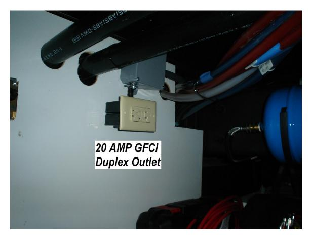
This GFCI outlet gets it power by using either shore power or generator power.
