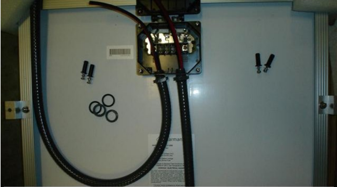
Added 125 Watt Panel 1
