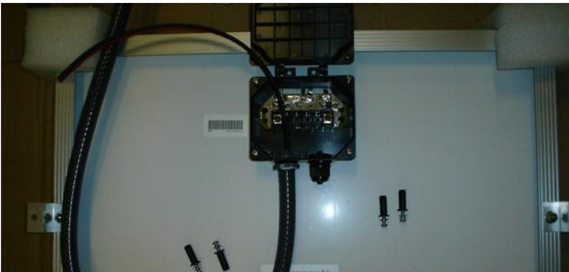
Added 125 Watt Panel 2
