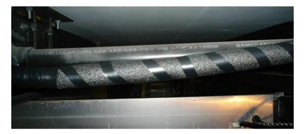
The final part of this modification was to insulate the water line cut-off valve and the water line on the back of the refrigerator as far up as I could reach to install the insulation.
