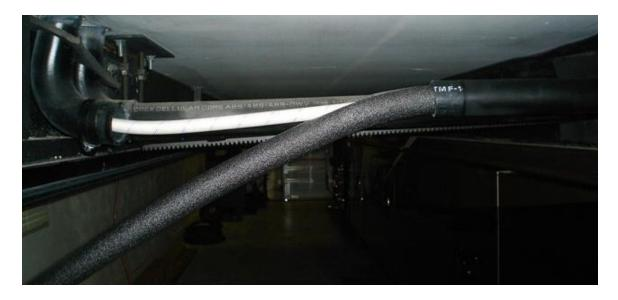
The worm gear pipe clamp securing the 1 1/2 inch ABS piping was loosened to access to the ice maker water line, which is a standard 1/2 inch white potable water hose. Tiffin used rubber radiator hose to route the water hose through the slide floor into the access behind the refrigerator. The IM water line was easy to insulate after cutting, the insulation was slid around the water hose then pushed into the ABS pipe about four feet.
