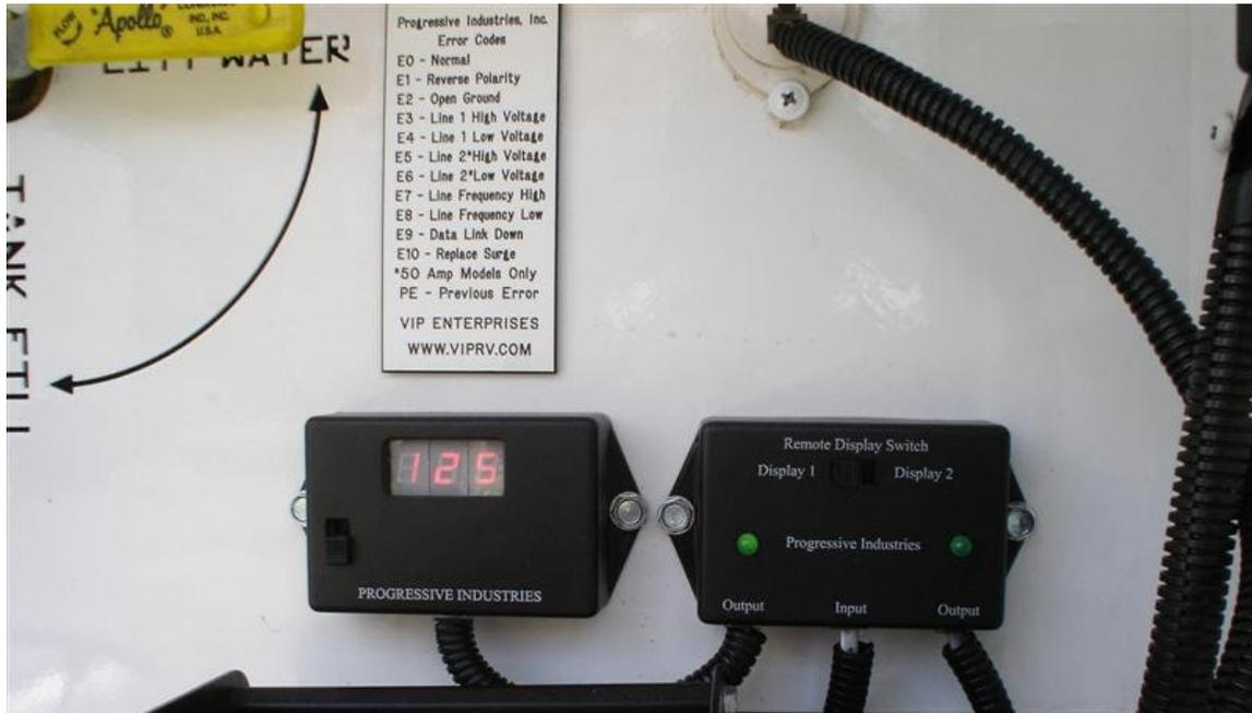
Or the inside display "Display 2". The coach's OEM telephone wiring was used to connect the Remote Display Switch to the inside "Display 2" as shown below. Shown below the display is located on the bedroom cabinet however this display could also be connected below the table or below the dash.
