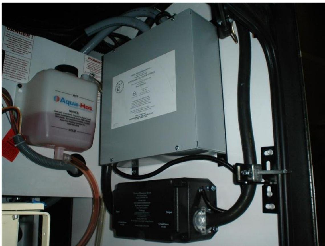
The incoming shore power cord was removed from the power transfer box. Enough slack cable was obtained in the shore power cord to mount the PI EMS-HW 50C box below the transfer box as shown in the above picture. The shore power cord was connected to the input side of the PI system. The output cord from the PI was pulled into the power transfer box where the
