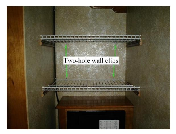
After installation the lower shelf is mounted six (6) inches above the wooden top of the electrical panel. The distance between shelves is thirteen (13) inches and the top shelf is about fourteen (14) inches below the closet's top wooden shelf.
