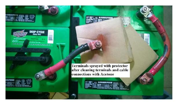
Two pieces of cardboard protect the batteries from overspray from the painting of the terminals with protector paint. Care is taken to make sure the terminal and cable connection are both well covered.
