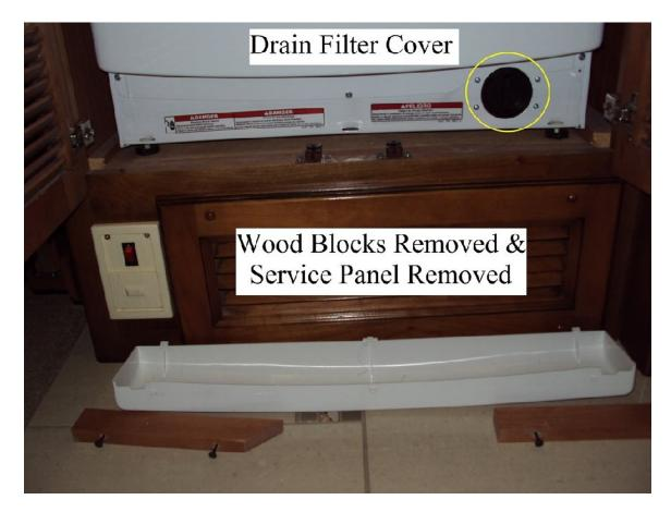
With the service panel removed the Drain Filter Cover is easily seen as noted by the yellow circle above.
