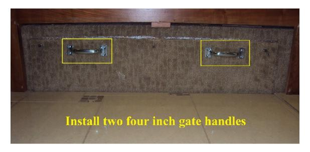
After the handles were installed it is easier to straddle the access cover, grab the two handles and pull back on them as you are lifting. You need to pull toward you to clear the lower closet trim as the cover is lifted. The forward lip of the cover has a metal lip which slides under the floor to prevent the front of the cover from lifting.
