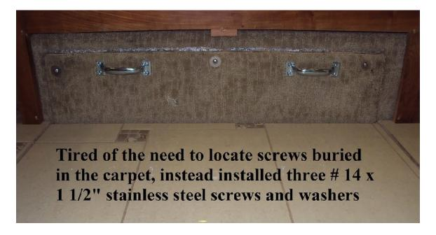
When it is time to re-install the cover the reverse operation works the best. Tuck the metal lip under the floor pull the cover toward you as the cover is
