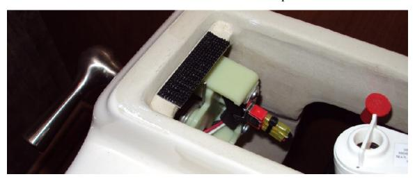
The first item, remove the lever using 1/8" Allen wrench, the screw is located under the lever. Second item, remove the three screws keeping the dump mechanism and switch mounted to the toilet.
