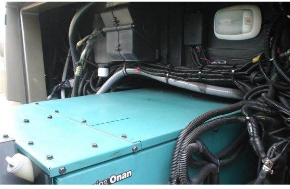
Rubber coated straps and tie wraps re-installed after firewall bare metal had been painted and installation of Crusingator's Modification # 50 - Dash AC Condensate Diverter had been installed.
