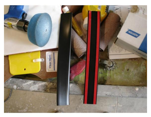
The two red protective strips are removed from the trim leaving an adhesive strip on the back which will stick the trim to the sidewall. The sealer filled sidewall cut is then straddled by the above trim strip.
