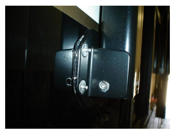
After sanding the pin flush with the pop rivet surface, a dab of clear silicone sealant was added over the pip hole for protection against any possible water entry around the pop rivets pin.
